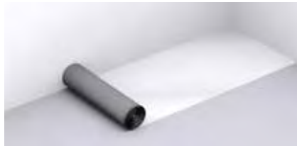
2. Extend the sheet in the longitudinal direction of the boards.
