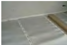
3. Overlap and seal with aluminum adhesive tape to give continuity to the insulation and prevent the passage of moisture.
