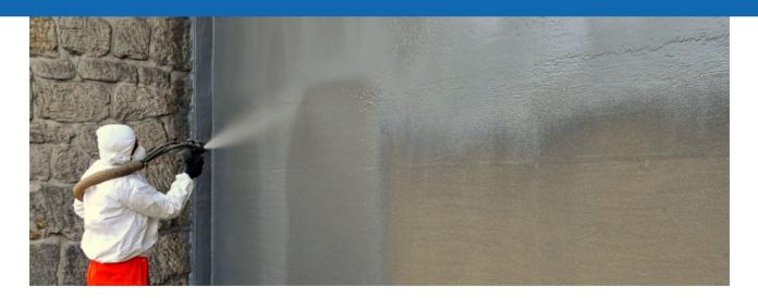
The **TIKIDAN Liquid Applied Waterproofing Membranes** are high performance waterproofing membrane, specially formulated and recommended for the most demanding waterproofing, protection and sealing jobs, both in new construction and in rehabilitation
